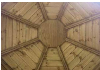
Internal roof structure
